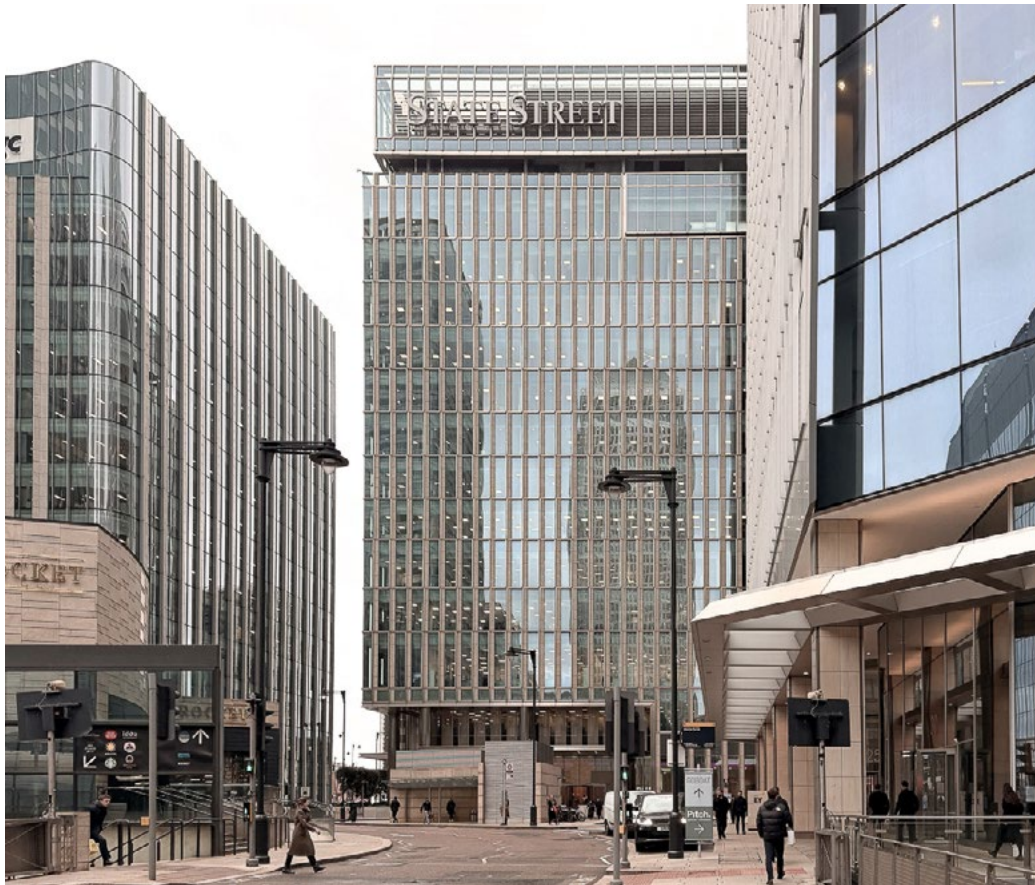
Existing view of 20 Churchill Place from Churchill Place (south)
